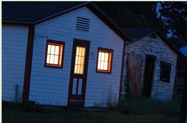
Renovated cabin and one needing improvements
